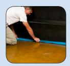
5 to 10 minutes. Any areas that dry prematurely should be sprayed again. Allow treated surfaces to dry before any additional procedures are initiated. After drying, remove any powdered residue using a stiff brush before continuing. At this point the floor can be polished and/or sealed. Polishing time will be reduced and less surface will absorb less sealer. Adjust procedures and/or applications appropriately.
