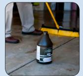
Spray section with water to determine if absorbency is consistent. This will also help you
